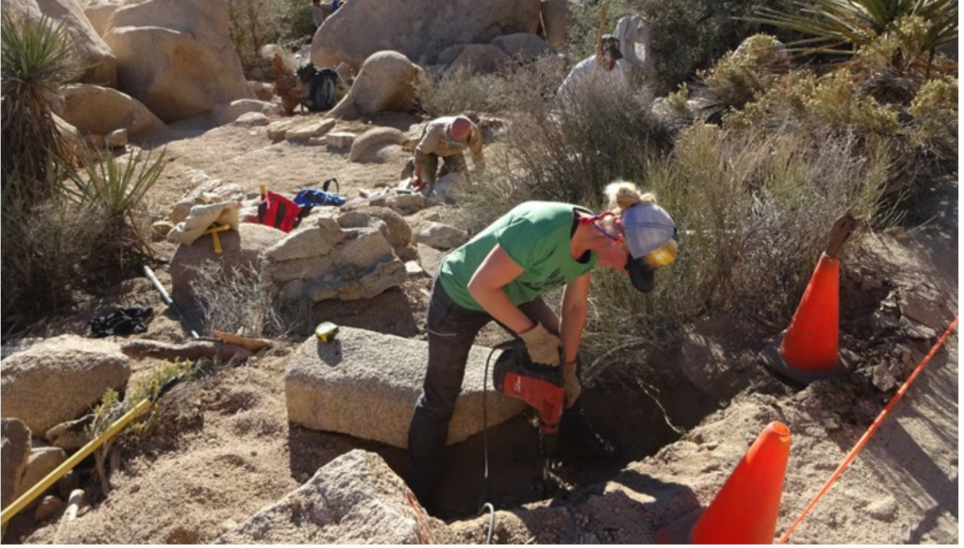
Amanda splits rocks to reconstruct the popular trail into Hidden Valley at Joshua Tree National Park. Ancestral lands of Serrano and Western Shoshone.
