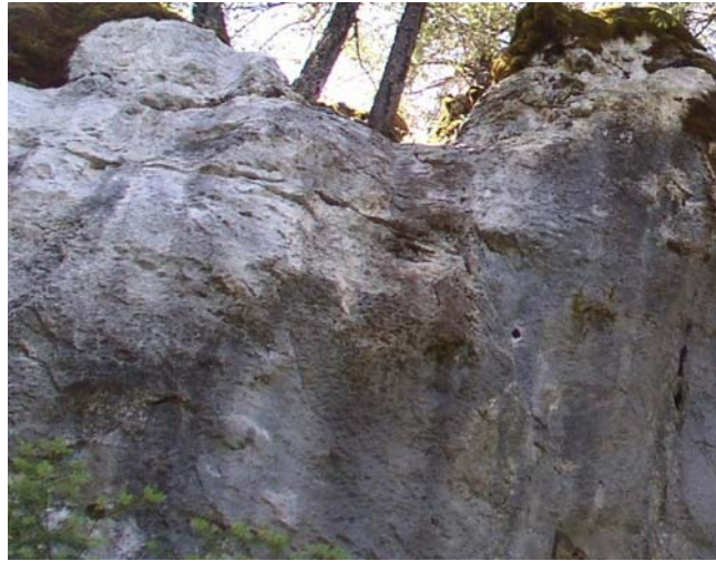
Climbing hardware and circular cut holes
