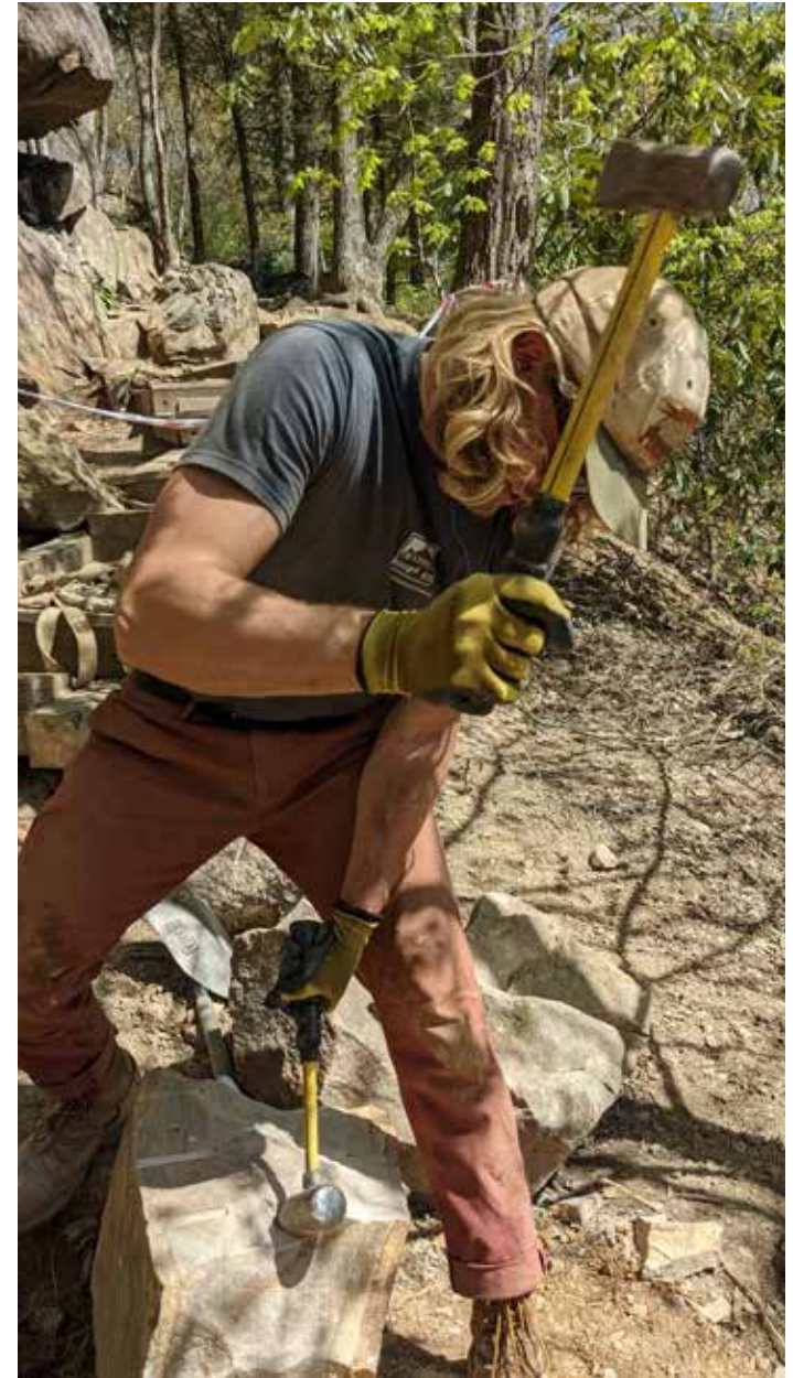
Conservation Team member Sam Richards splitting rock for a stone staircase, Bridge Buttress, New River Gorge, West Virginia, ancestral lands of S'atsoyaha, Tutelo and Moneton. © Access Fund.
